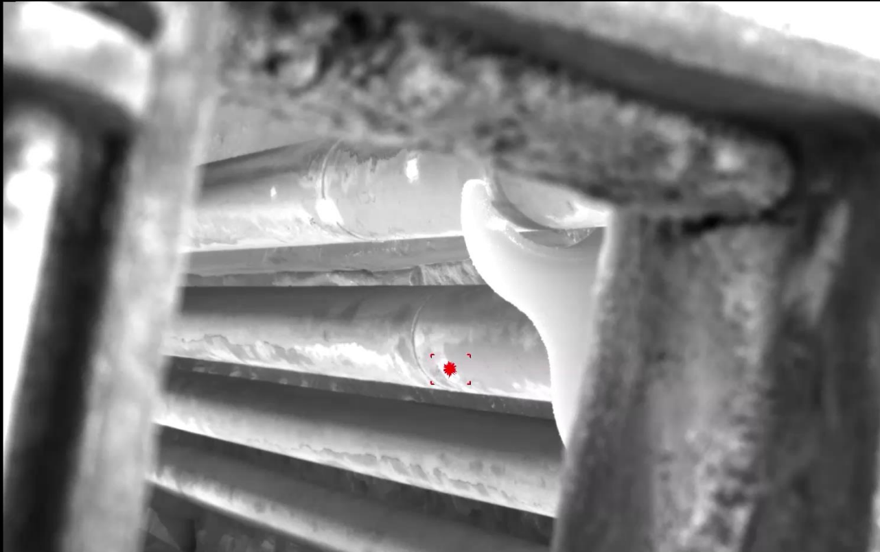
Petrochemical furnace: T air: 980°C – T pipe: 580°C
